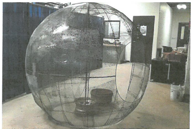
Mesh applied for fiberglass attachment supports
